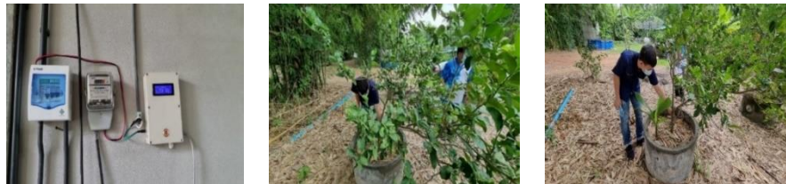
Figure 3. IoT-CLP system installation in Maha Sarakham Province
