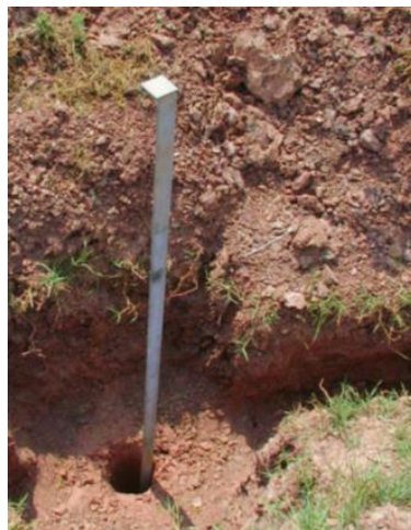
Figure 2. Vertical Ground Electrode Grounding System
