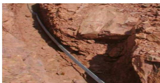
Figure 3. Horizontal Ground Electrode Grounding System
