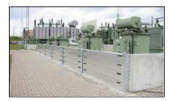
Figure 3. Floodwall protection using concrete walls and removable panels [4]
