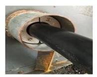
Figure 4. Use of seal for the cable entry hole
