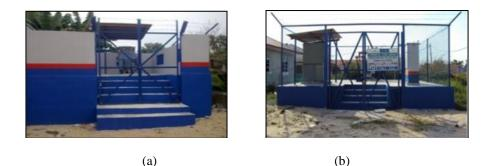
Figure 2. (a) Raised substation for flood level above 3 metres (b) Raised substation for flood level below 3 metres
