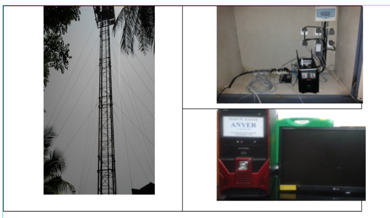
Figure 4. Anyer Radar Station
