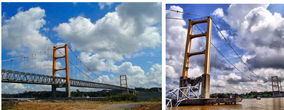
Figure 2. Kutai Kartanegara Bridge before and after collapse [7]
