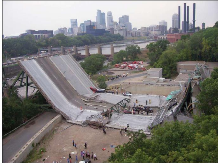
Figure 1. One section of the I-35W Bridge collapse [6]
