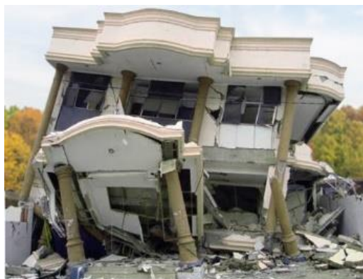
Figure 1. The building sink due to liquefaction
