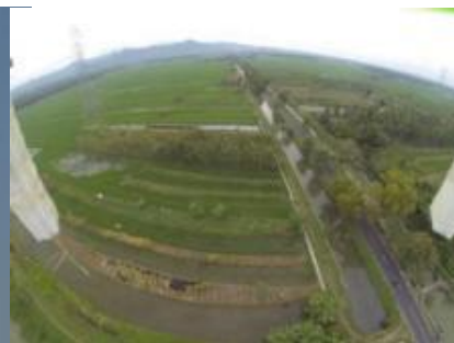
Figure 16. Aerial photos viewed from south side to the new airports
