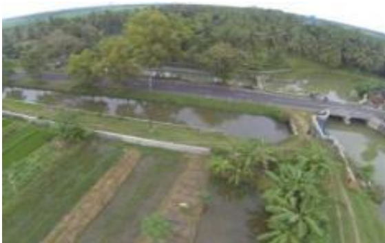
Figure 19. West to the gate 35 meters above ground level
